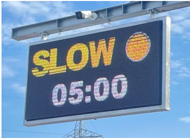
2. Figure: Technical failure
