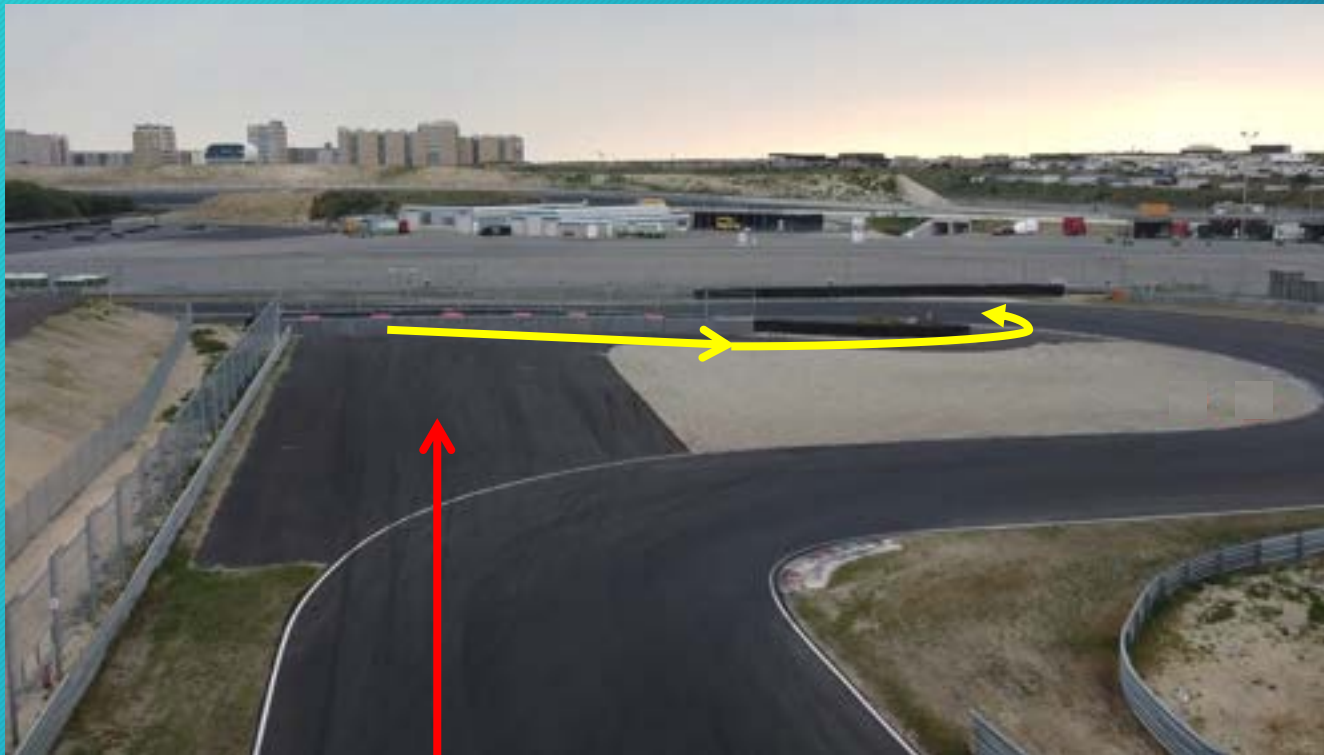
Asfalt run off area
